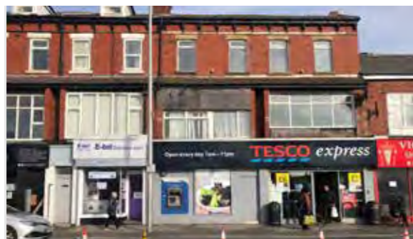
Type 3 - 1st and 2nd Floor HMOs on Central Drive
